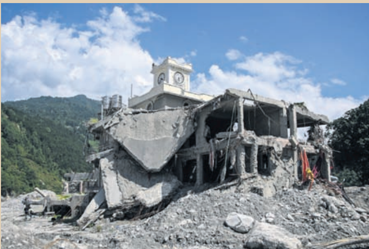
A general view shows damaged houses in the aftermath of the August 26 flash flood at Betrawati in Nepal's Nuwakot district on October 1, 2026.
