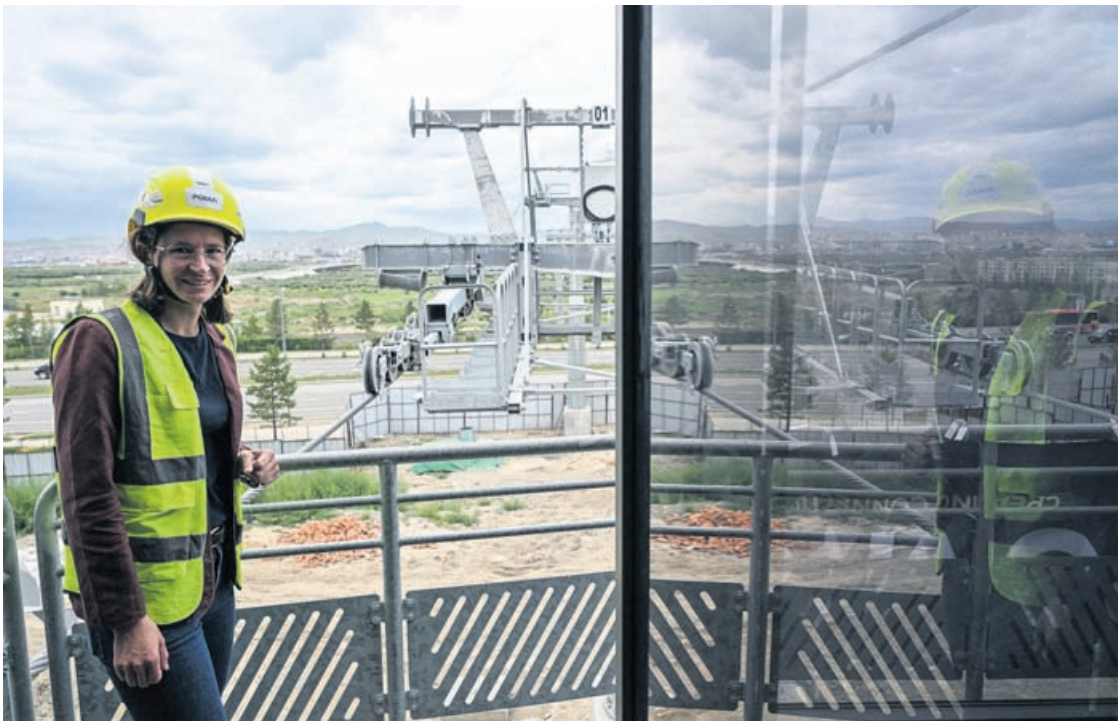
Project manager Cecile Broi looks on during an interview at the site an under construction cable car led by French firm Poma in Ulaanbaatar on August 22, 2026.
