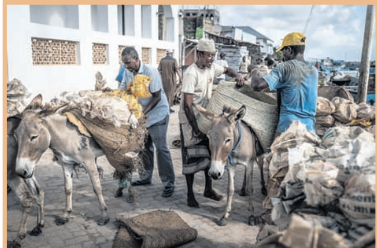
Workers load construction materials onto donkeys for transport at the seafront in Lamu Old Town on Lamu Island on October 1, 2026.
