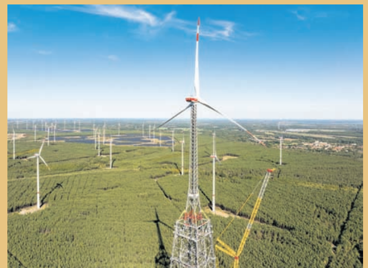
27 September 2026, Brandenburg, Schipkau: The wind tower in Schipkau already towers over neighboring wind turbines (aerial view taken with a drone.)
