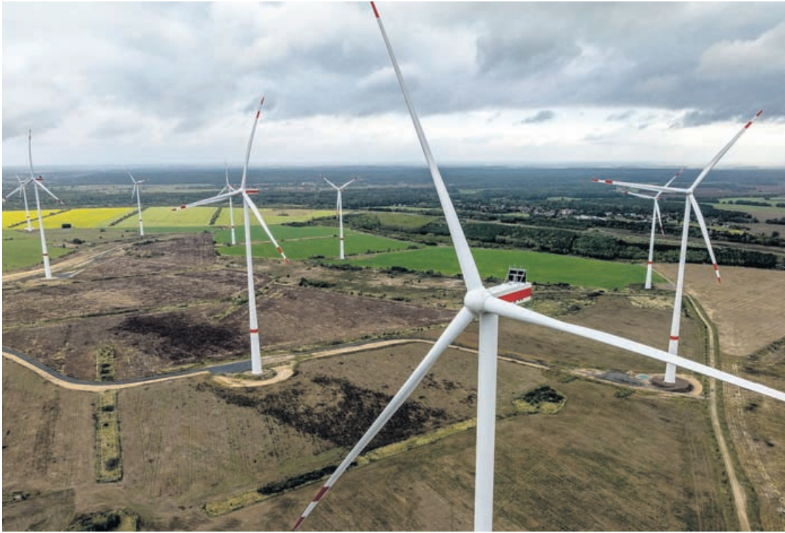
Wind turbines spin at the Briesnig II wind farm on the site of the former Jänschwalde open-pit mine (aerial view taken with a drone).
