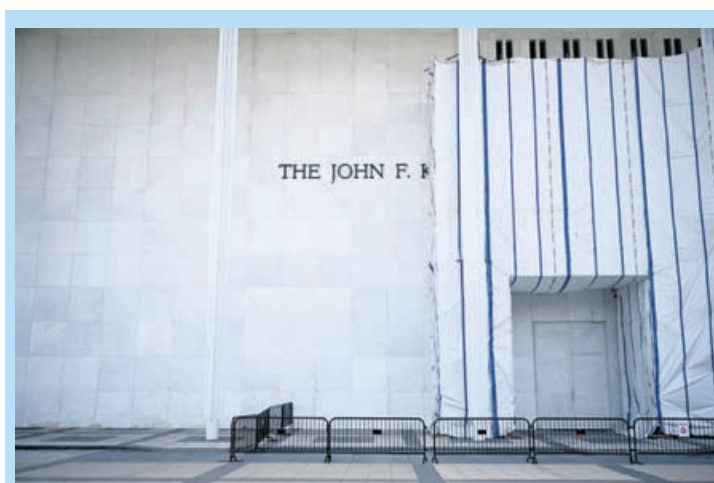
Scaffolding and a large protective tarp is covering part of the facade of the John F. Kennedy Center for the Performing Arts in Washington, DC, on August 13, 2026.
