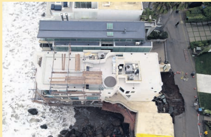
This aerial view shows a sinkhole on a street and driveway of a seaside home affected by large swells produced by Hurricane Marie in Malibu, California, on September 8, 2026.
