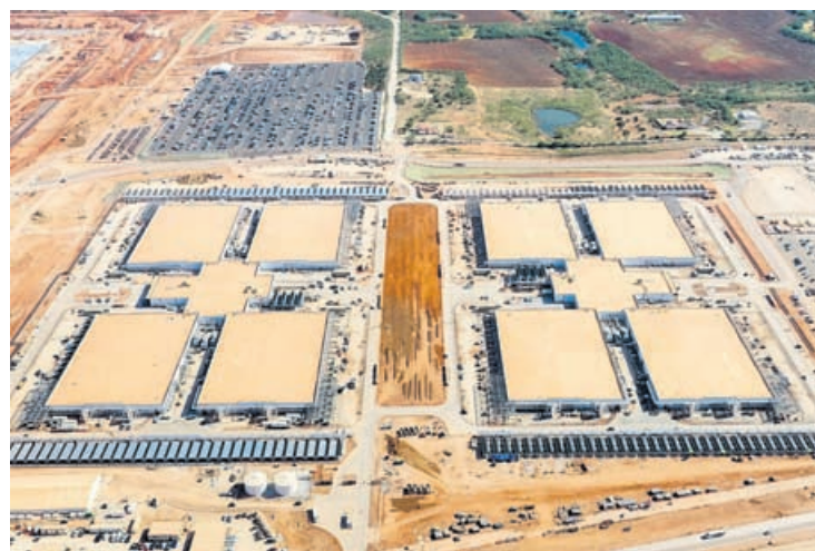
In an aerial view, the Stargate Oracle AI data center campus is seen on August 26, 2026 in Abilene, Texas.
