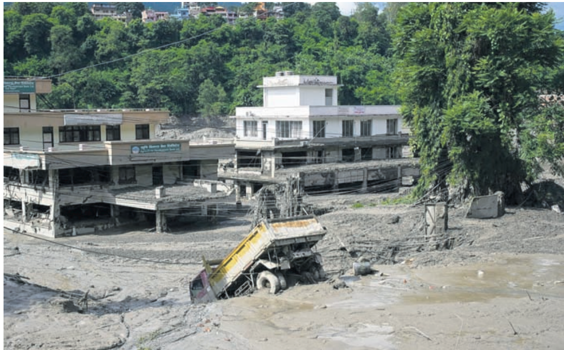
A photograph taken on August 26, 2026 shows a truck and buildings partially submerged by mud after flash floods and a landslide in Trishuli Bazar, in Nepal's Nuwakot district (Prakash Mathema/AFP/Getty Images)
