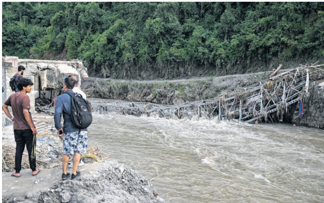
People stand near a collapsed bridge after flash floods at Devighat in Nepal's Nuwakot district on August 28, 2026.
