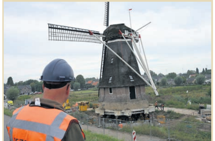
Workers take part in the lifting operation of a 250-year old windmill in Waardenburg on August 28, 2026.
