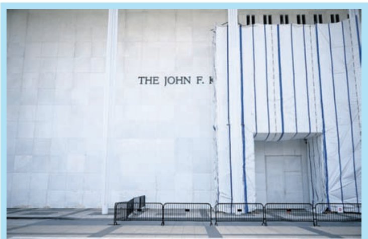
Scaffolding and a large protective tarp is covering part of the facade of the John F. Kennedy Center for the Performing Arts in Washington, DC, on August 13, 2026.
