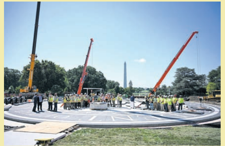
Workers look on at the construction site of a helipad as US President Donald Trump speaks to the press on the South Lawn of the White House in Washington, DC, on August 19, 2026.
