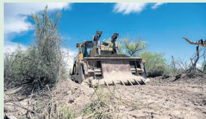
Heavy machinery is seen inside Big Bend National Park in southern Texas, on August 15, 2026.
