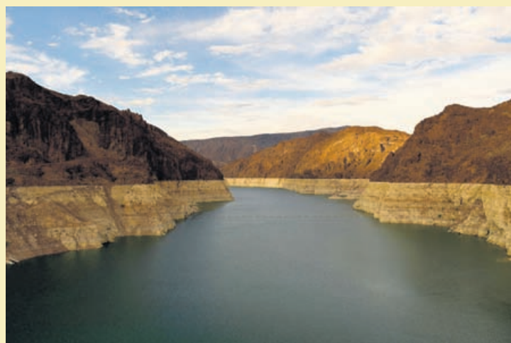
A "bathtub ring" is visible at sunset during low water levels the Lake Mead reservoir due to the western drought on July 19, 2021 as seen from the Hoover Dam on the Colorado River at the Nevada and Arizona state border.
