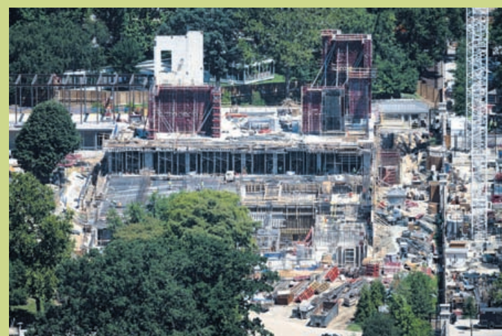
A view of the ongoing construction of a planned ballroom at the White House, as seen from the Washington Monument observation deck in Washington, DC on July 23, 2026.
