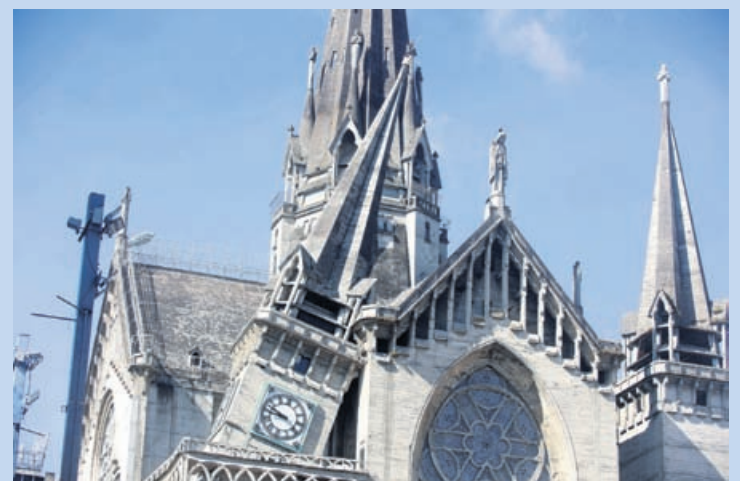
The damage sustained by the Manizales Cathedral are pictured after the earthquake in Manizales, Colombia, on August 10, 2026.
