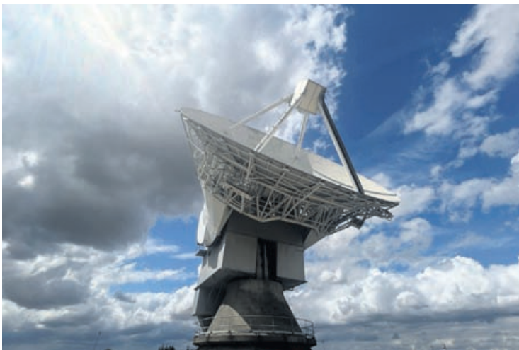
This photo taken on July 30, 2026 shows the antenna dish installation at Chilbolton Observatory in the village of Chilbolton, south-west of London.
