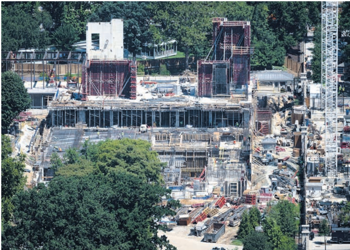
A view of the ongoing construction of a planned ballroom at the White House, as seen from the Washington Monument observation deck in Washington, DC on July 23, 2026.
