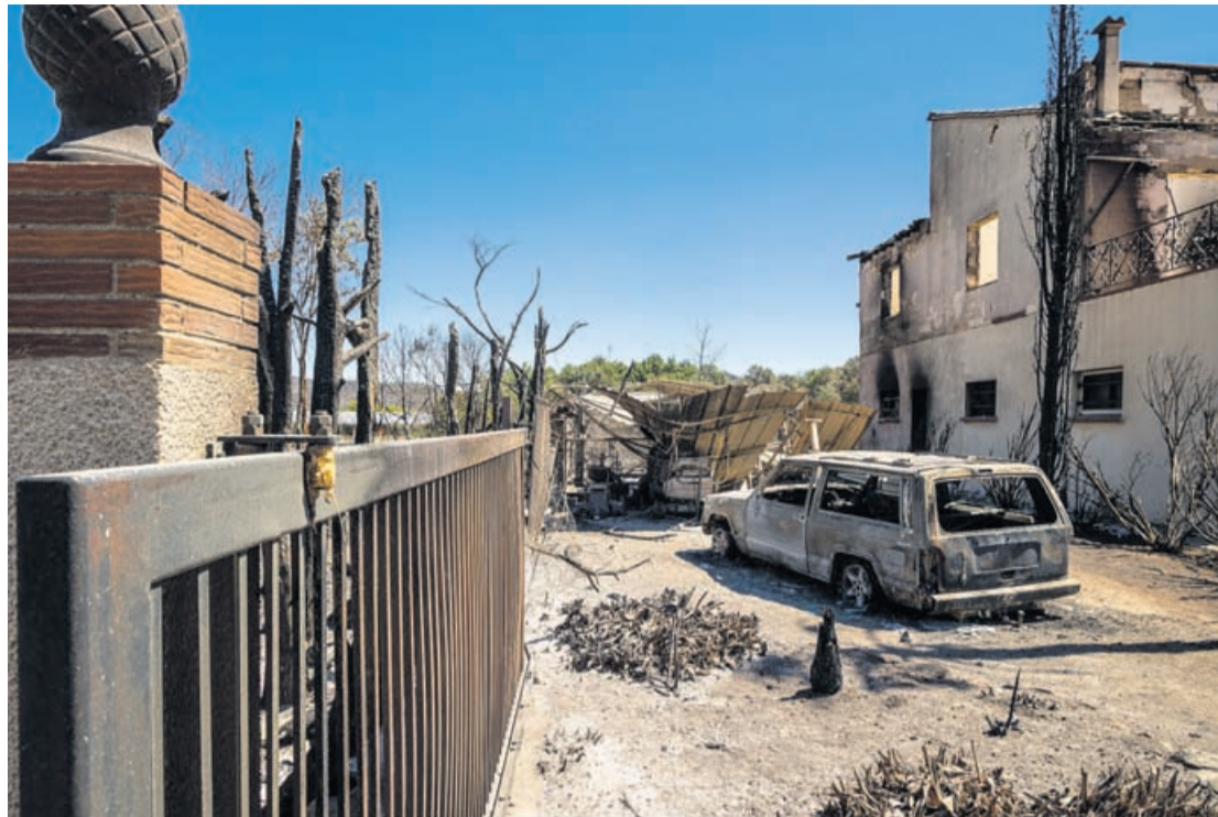
This photo shows a house destroyed by fire in Rodes on the outskirts of Ille-sur-Têt, in the Pyrénées-Orientales department in the south of France on July 7, 2026.
