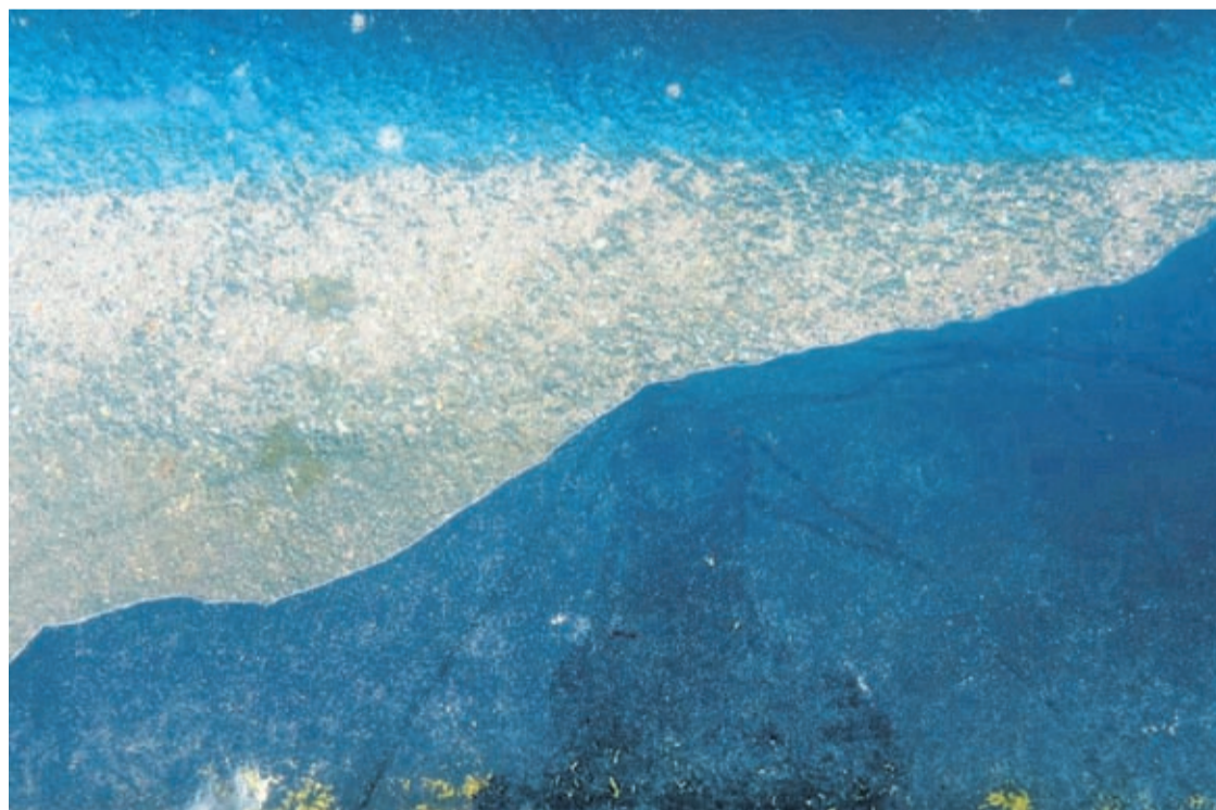
Paint peels away from the bottom of the Lincoln Memorial Reflecting Pool, in Washington, DC, on June 23, 2026.
