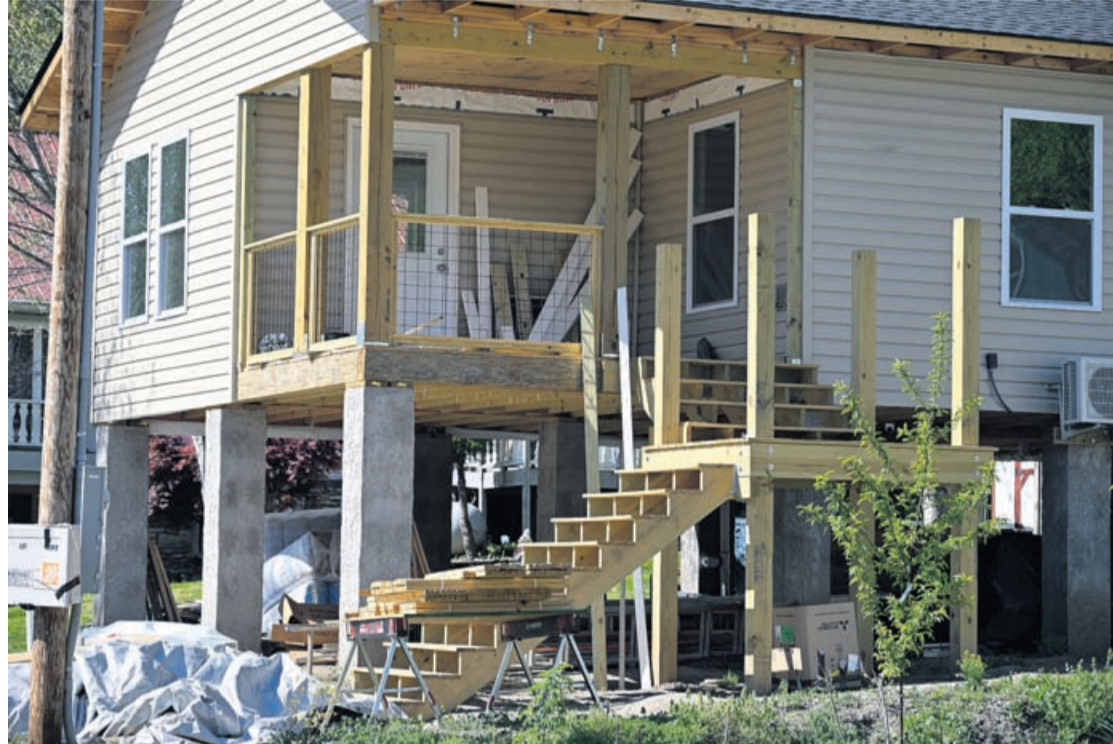
Homes under construction in Marshall, North Carolina, on April 9, 2026.
