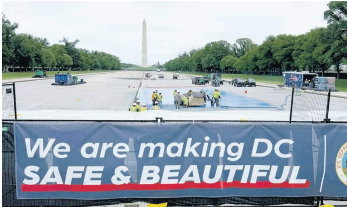
Crews resurface the bottom of the Lincoln Memorial Reflecting Pool with a new blue coating in Washington, DC on April 25, 2026.
