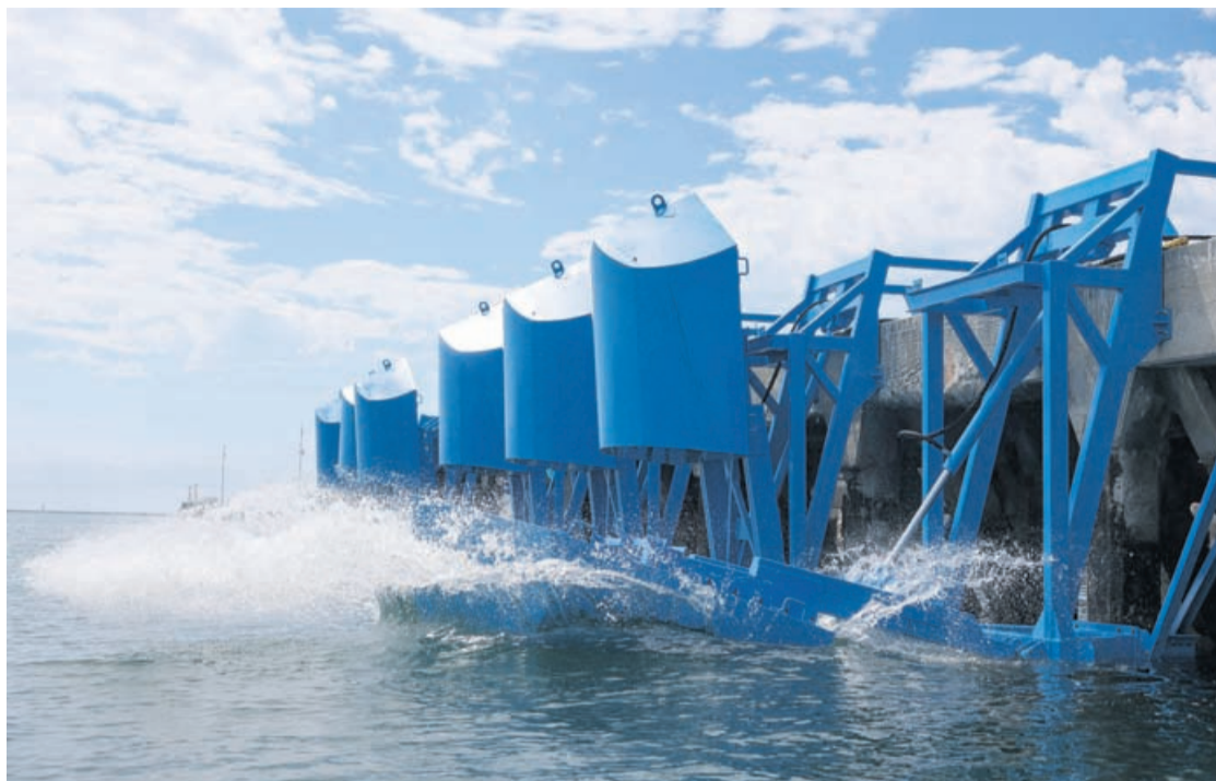
Floaters are released into the water during a demonstration of Eco Wave Power electricity generation technology using the power of ocean waves in the harbor at AltaSea at the Port of Los Angeles in San Pedro, California, on August 26, 2025.
