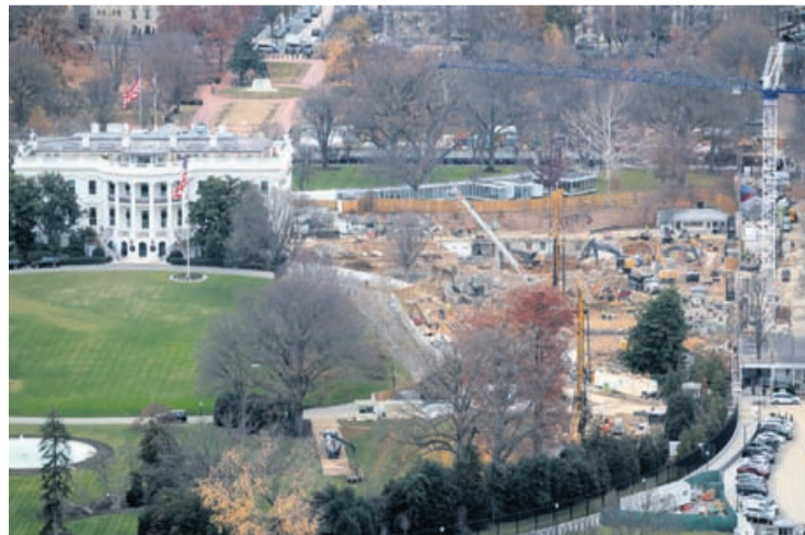
Demolition work continues where the East Wing once stood at the White House on December 8, 2025 in Washington, DC.
