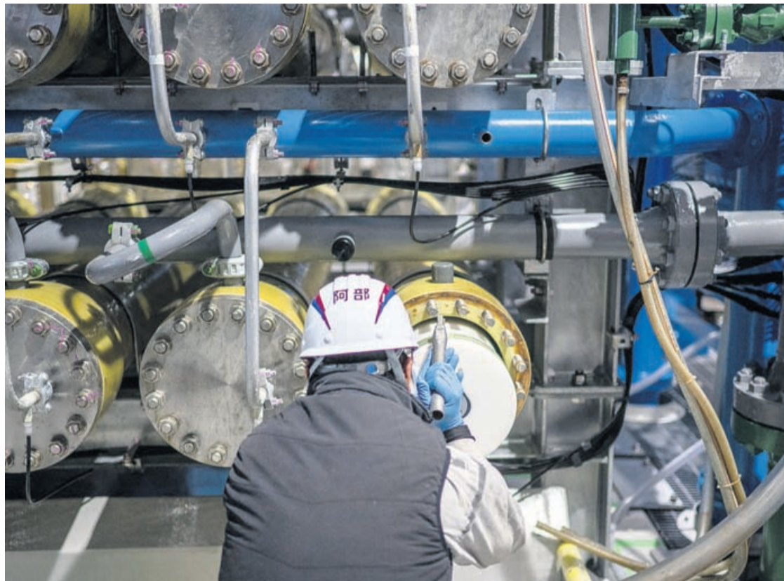
This picture taken on January 14, 2026 shows a staff member changing a part of the osmosis membrane facilities at Sea Water Desalination Plant in Fukuoka.
