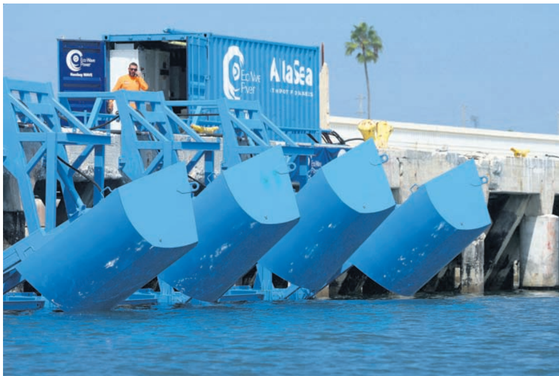
Floaters are raised out of the water during a demonstration of Eco Wave Power electricity generation technology using the power of ocean waves in the harbor at AltaSea at the Port of Los Angeles in San Pedro, California, on August 26, 2025.
