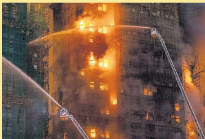
Firefighters try to extinguish a flames engulfing a building after a fire broke out at Wang Fuk Court, a residential estate in the Tai Po district of Hong Kong's New Territories, Wednesday, Nov. 26 2025.
