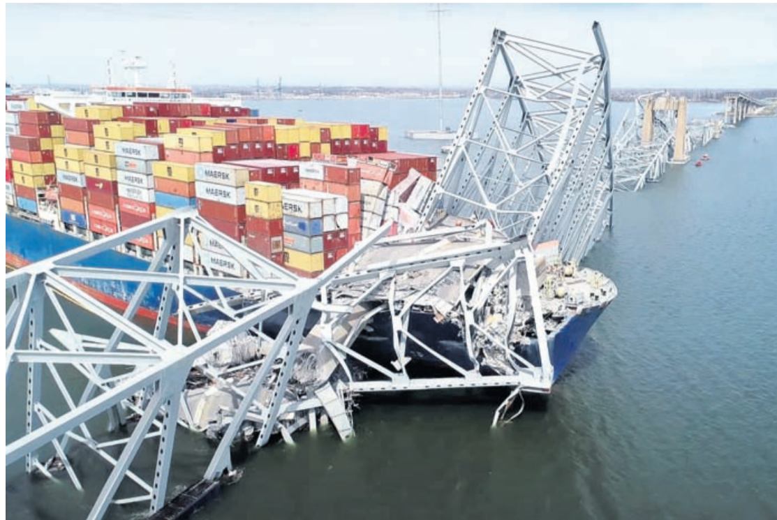
In this image taken from video released by the National Transportation and Safety Board, the cargo ship Dali is stuck under part of the structure of the Francis Scott Key Bridge after the ship hit the bridge, Tuesday, March 26, 2024, in Baltimore.
