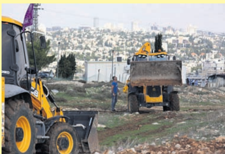
In this Nov. 16, 2020 file photo, workers take a break before European Union officials visit the construction site for the Givat Hamatos Israeli settlement, in Jerusalem.
