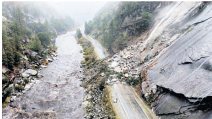
Rocks and vegetation cover Highway 70 following a landslide in the Dixie Fire zone on Sunday, Oct. 24, 2021, in Plumas County, Calif.
